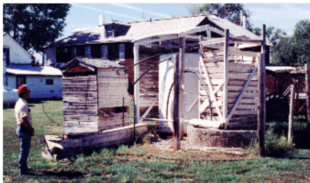
Figure 2. Storage tank and cooling tower for the Stoppel Hotel.
