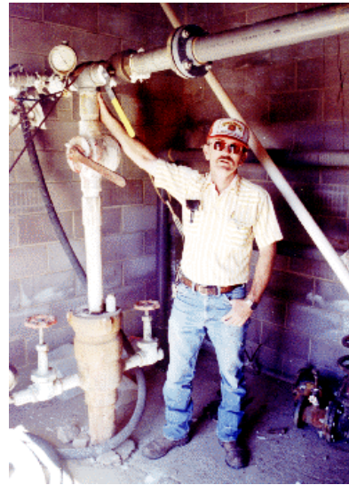
Figure 4. Geothermal well with Ruben Vollmer.
