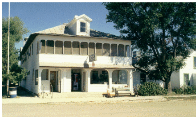
Figure 1. The Stoppel Hotel with the bath area on the right.
