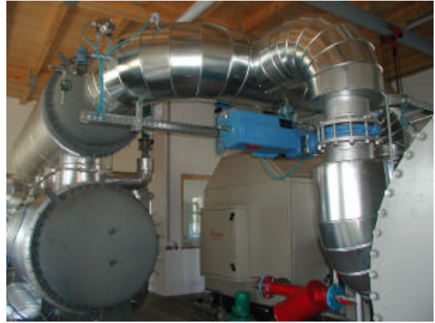
Figure 6. ORC generator.
