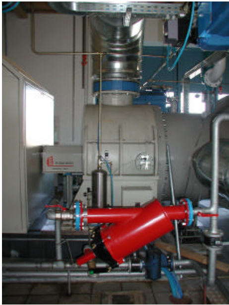
Figure 5. ORC turbine.
