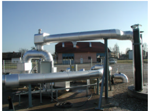
Figure 4. Well 1A with pump house.
