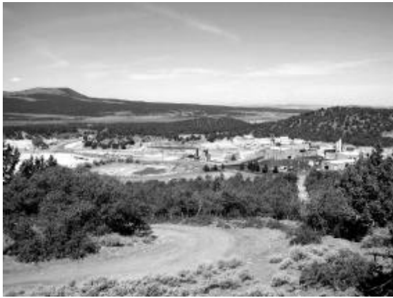
Figure 8. Overview of the power plant. The sulfur deposit and Cove Fort volcano are in the background.
