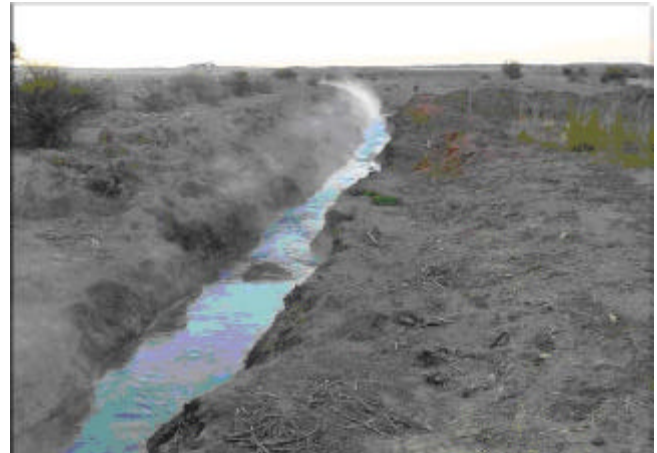
Figure 5. The outlet water from the power station is flowed in a channel until it has cooled sufficiently for use by stock animals (Australian Broadcasting Corporation).
