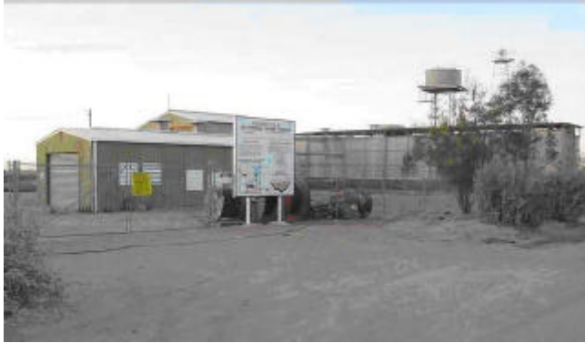
Figure 3. The Birdsville Geothermal Power Station is situated on a free flowing bore a mile or so out of town (Australian Broadcasting Corporation).
