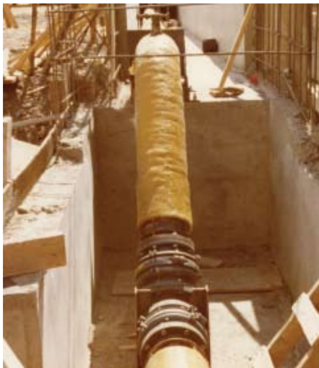
Photo 3: Production Pipeline and Tunnel Construction (Babcock)
