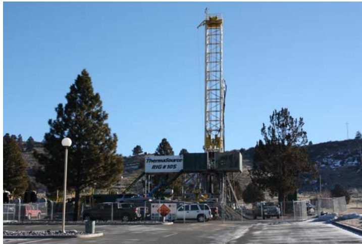
The drilling rig being set-up.
