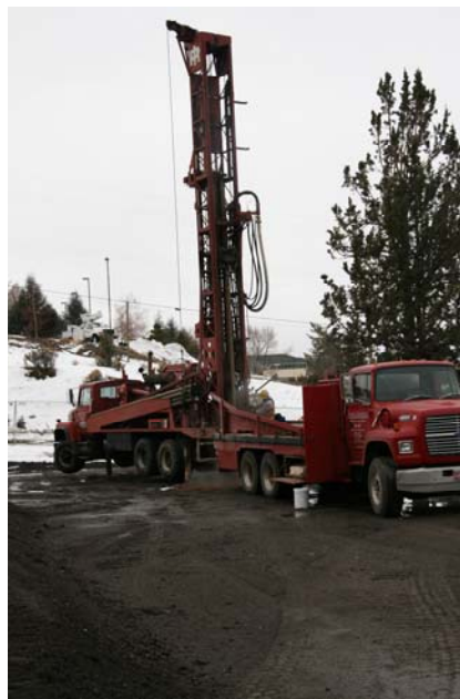
Start of drilling for surface casing.
